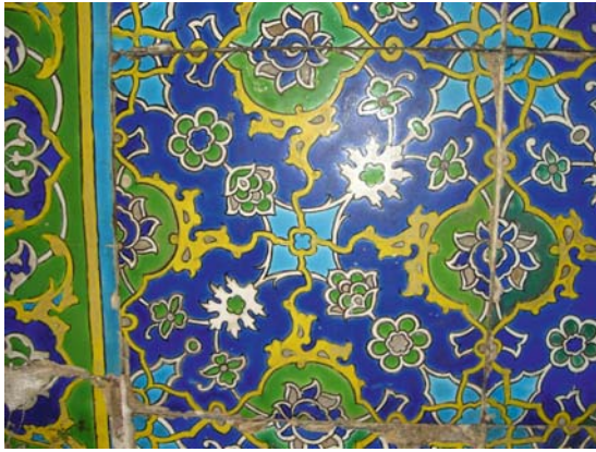
Architectural Decoration in Islam: History and Techniques. Fig. 16 Detail of cuerda seca tiles currently embedded in a re-constructed wall in the Topkapi Palace. Istanbul, Turkey. Late fifteenth century.
